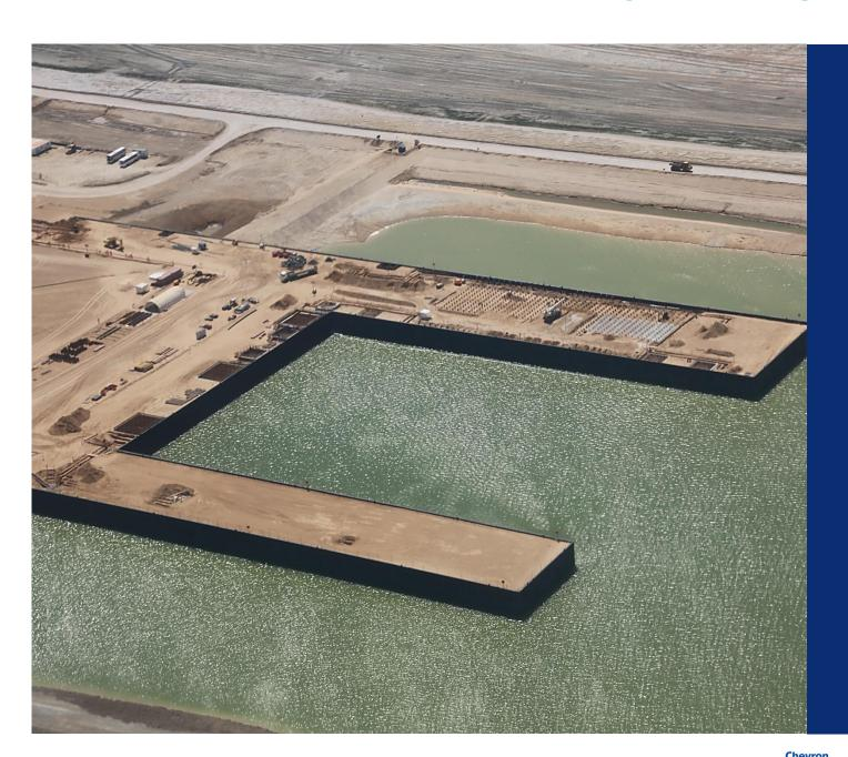
Marine channel, excavation of nearshore channel and controlled flooding of the turning basin
