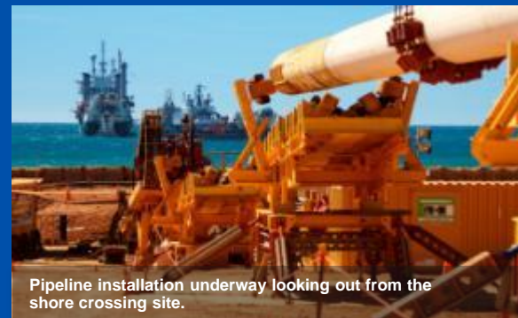
Directionally drilled shore crossing site on Barrow Island
