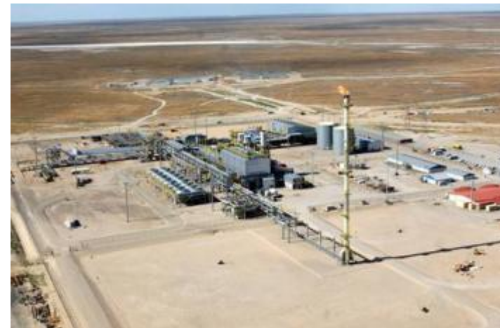
SGI facilities: replicated with FGP
