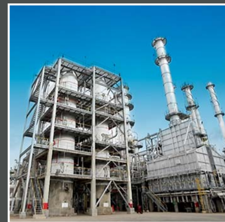
Lube Oil Plant
