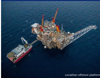
Leviathan offshore platform
