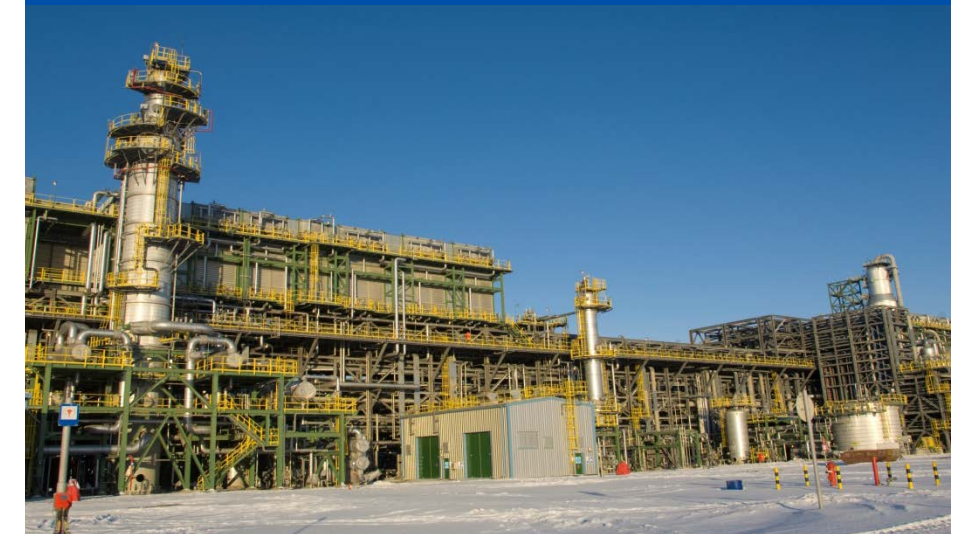
WPM – Wellhead Pressure Management SGP – Second Generation Project FGP – Future Growth Project
